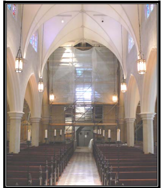
VIEW OF REAR GALLERY UNDER CONSTRUCTION
